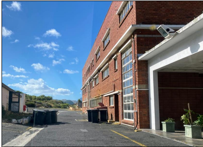
Figure 7. Empty waste bins after waste collection at Job Maseko. The bins will be stored in the outbuilding on the left.
