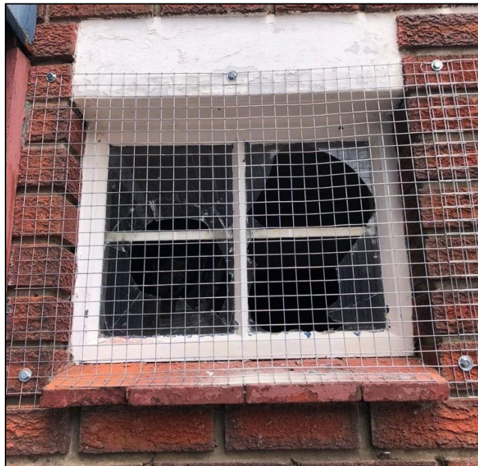
Figure 8. Newly secured windows at West Yard.
